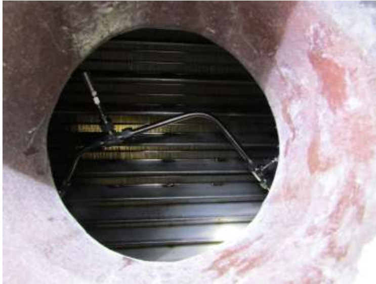
Fig.11. View Through Bottom Sight Glass Port Showing Diffuser Piping and Johnson Screen
